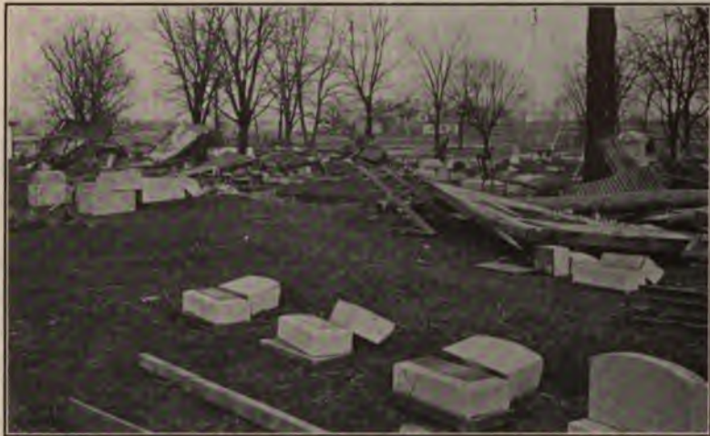
FIG. 32.—Although the velocities in the 1913 Ohio flood were sufficient to overturn tombstones, yet the sod prevented erosion.
